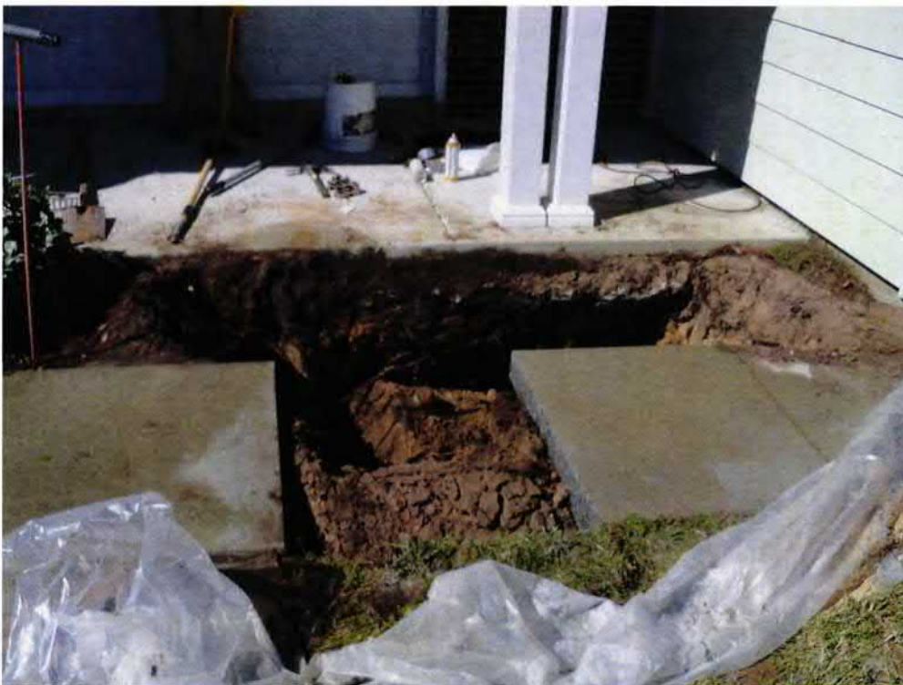
Picture 2: UST 210Balsam excavation.
